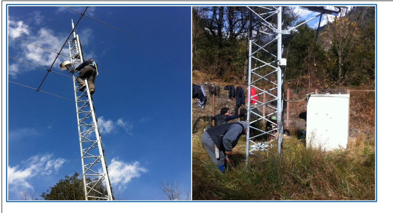
Pic 9: Realignment of DCP for EUMETSAT from Meteosat-7 at 57 ° to Meteosat-8 at 41.5 °.
