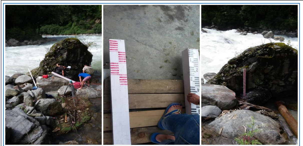
Pic 15: Water Level Guage Installed for Gasa Dzongkhag.
