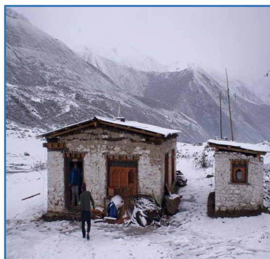
Pic 4: Renovated Flood Warning Office
