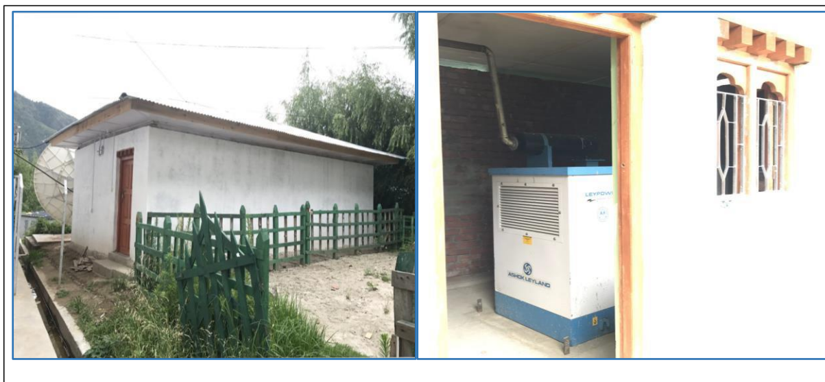
Pic 12: Generator Shed Constructed at NFWFC, Thimphu
