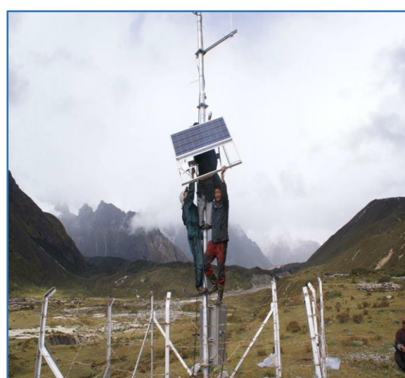
Pic 6: Repairing of Solar Panel at Lunana
