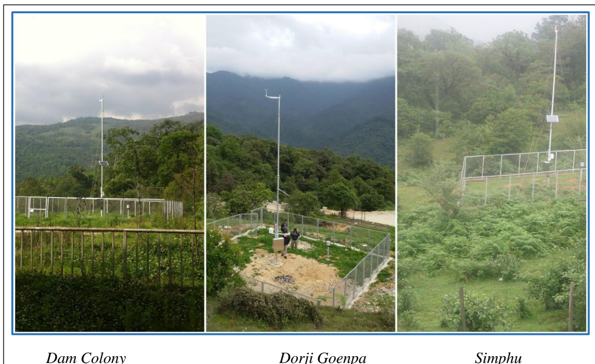
Pic 10: AWS installed in Mangdechhu sub-basin
