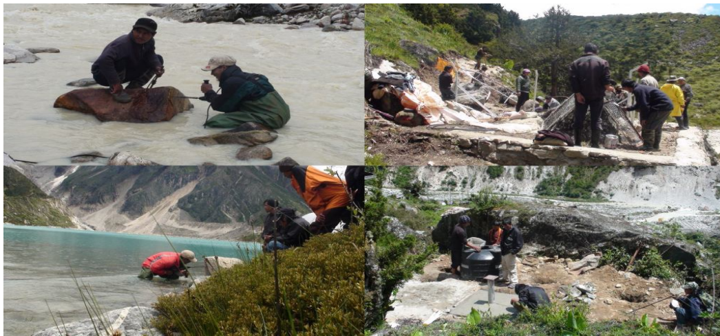
Photo 20: Progress of civil works in Lunana (August 2011)
