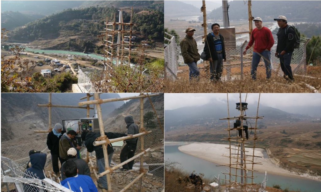
Photo 18: Installation of Sirens in Punakha-Wangdeu valley (January 2011)
