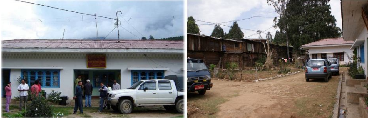
Photo 4: Wangdue Flood Warning Office
