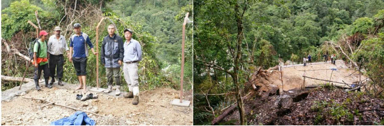
Photo 11: Progress of civil work at Dangsa for Automatic Water Level Site above Tamedamchhu, Punakha (August 2010)
