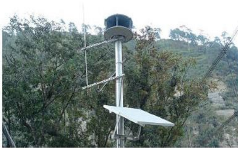
The early warning flood siren at Kamichhu, Wangdue
