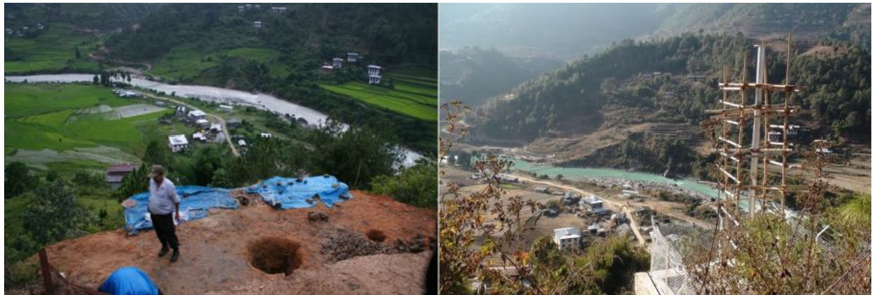
Photo 12: Progress of civil work at Samdingkha Siren Station (August 2010)
