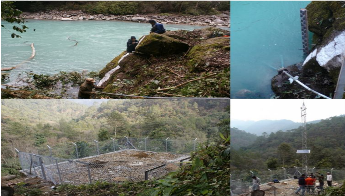
Photo 17: Installation of AWLS at Dangsa, Tame Damchhu (January 2011)
