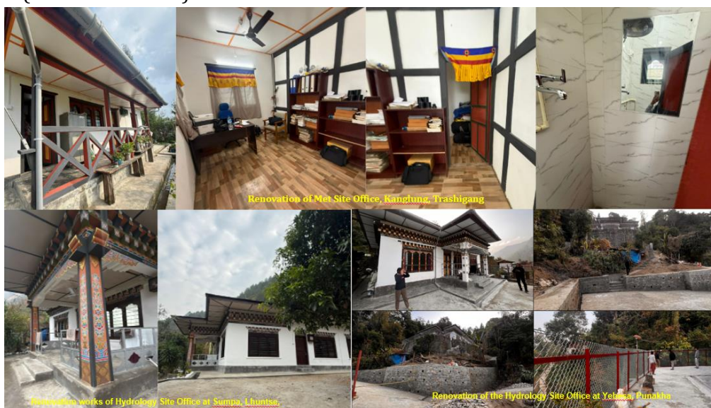
Figure 27:: Renovation of Site Offices and Laboratories under GoI-FWS and RGoB support
