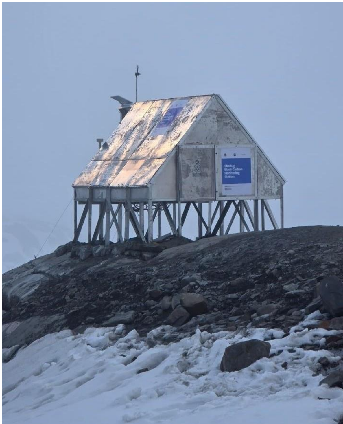
Figure 9: Bhutan's First Black Carbon Monitoring Station on Shodug Glacier (Headwater of Thimchu) installed under NCHM-ICIMOD Partnership
