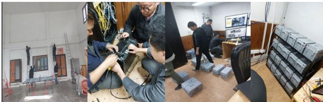
Figure 32: Photos from Installation of UPS at Paro International Airport (PIA)
