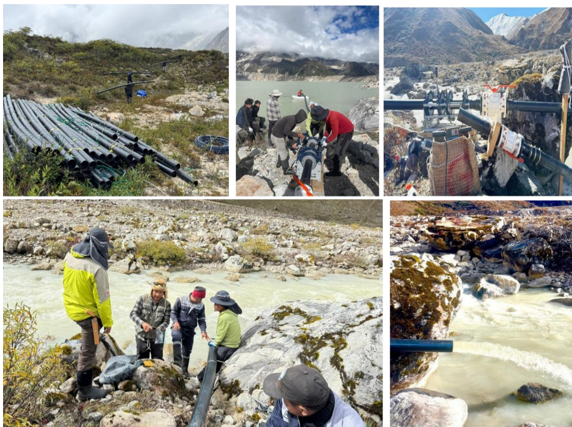
Figure 50: Photos NCHM conducting test siphon and bud-fusion joining of HDPE pipes at Thorthormi Lake site
