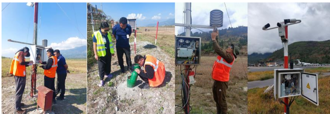
Figure 34: Photos from Annual Maintenance at international and domestic airports
