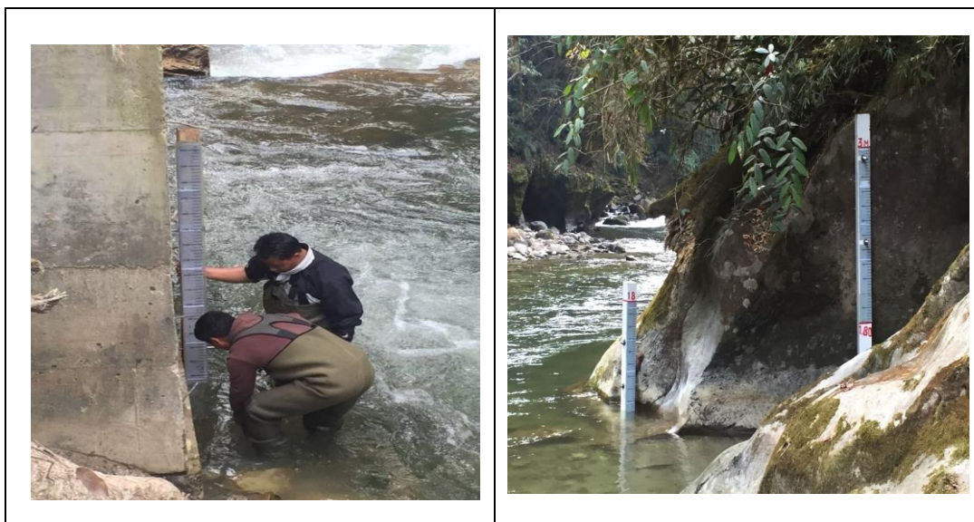
Figure 57: River Gauge Post being installed at Nikachhu near Bailey Bridge
