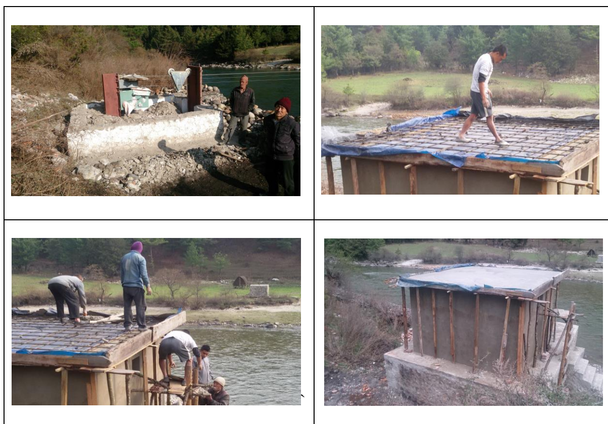
Figure 3: The existing cableway at Kurjey, Bumthang raised by 1.7 M to avoid the flooding of the station during the flood.
