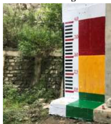
Figure 3: Water level marking at Dechencholing-Taba Bridge with Normal (Green), Alert (Yellow) and Alarm (red) water level
