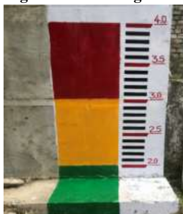
Figure 3: Water level marking at Dechencholing-Taba Bridge with Normal (Green), Alert (Yellow) and Alarm (red) water level
