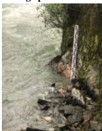
Figure 3: Water level marking at Dechencholing-Taba Bridge with Normal (Green), Alert (Yellow) and Alarm (red) water level
