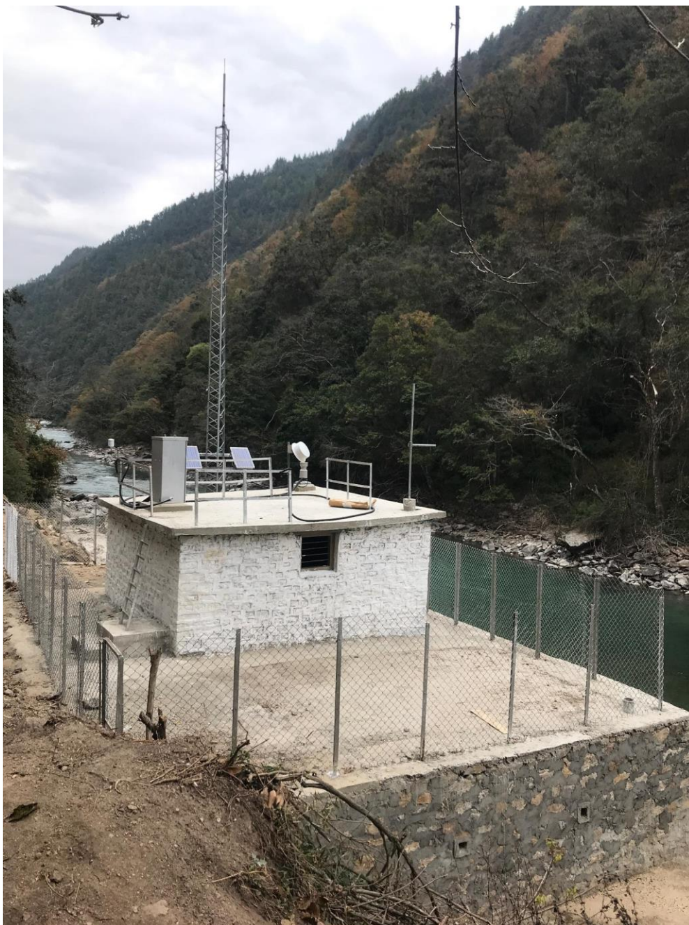
Figure 1: Rehabilitated Bjizam Hydrological Station with Automatic Water Level Station (AWLS), and Communication system for Flood EWS on Mangdechhu (October, 2022)
