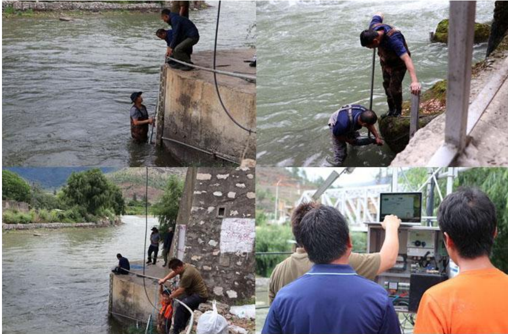
Figure 49: Installation of WQMS at Parochhu
