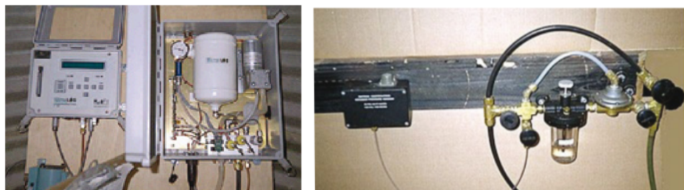
Figure 2: gas-purge system
