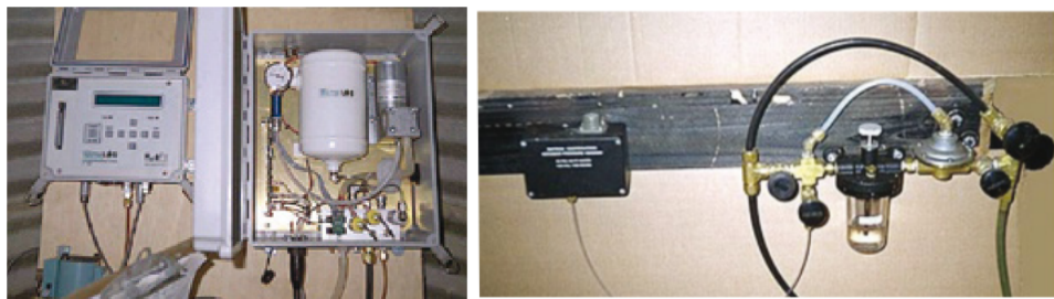
Figure 2: gas-purge system
