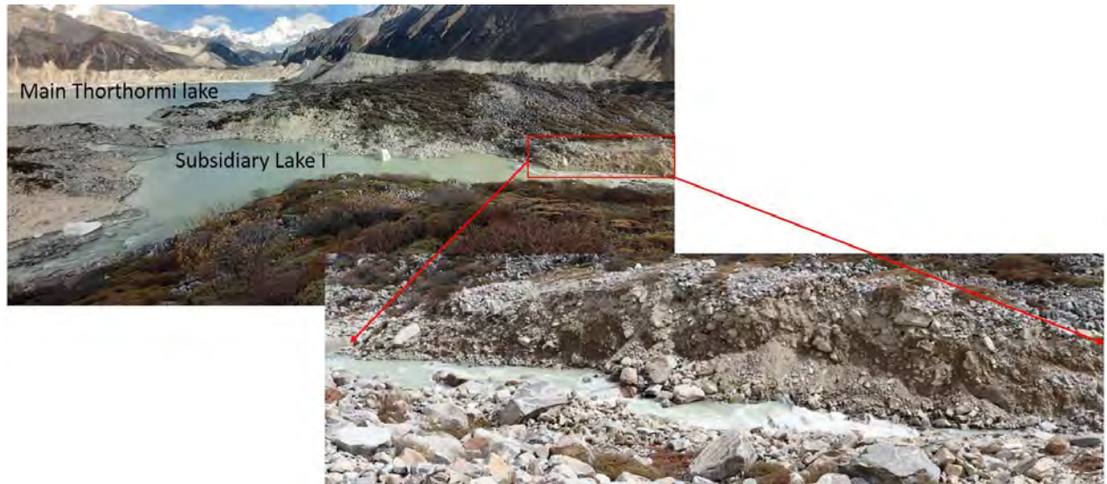
Photo 6: Erosion and scouring in the channel between subsidiary lake I and subsidiary lake II
