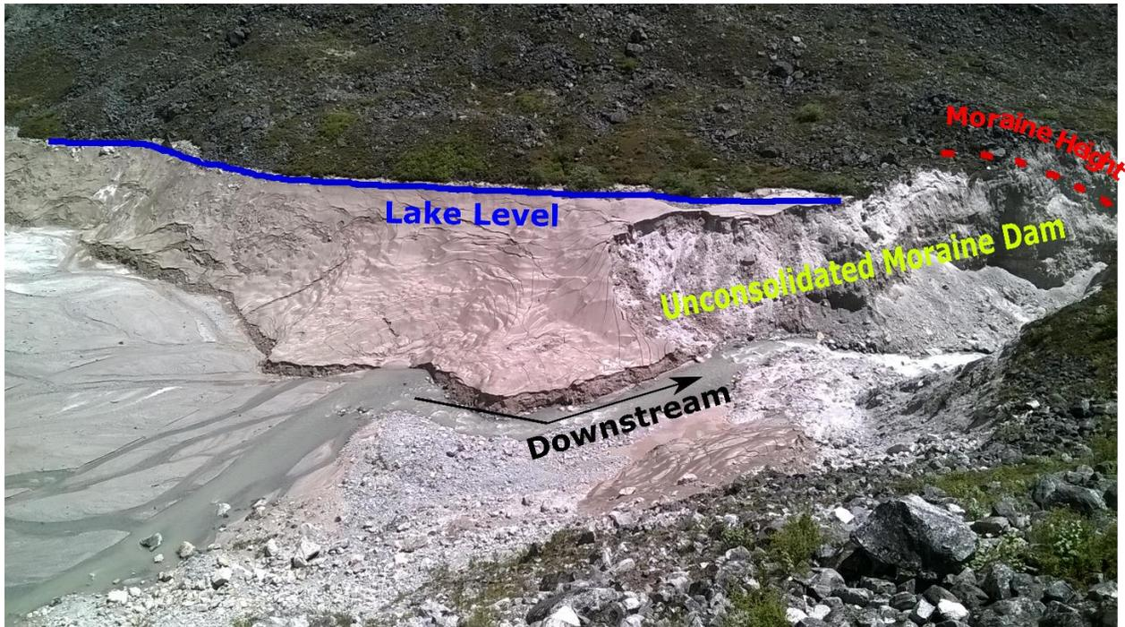
**Figure 3.2:** Remnants of Lemthang Lake after the GLOF. Blue line shows the original Lake level and the dotted red line shows the original moraine dam height near the outlet.
