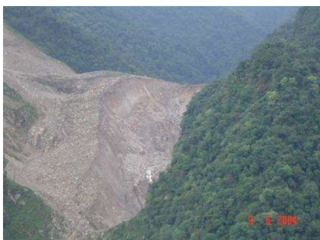
Figure 3: Tsatichhu Landslide Dam (2003)
