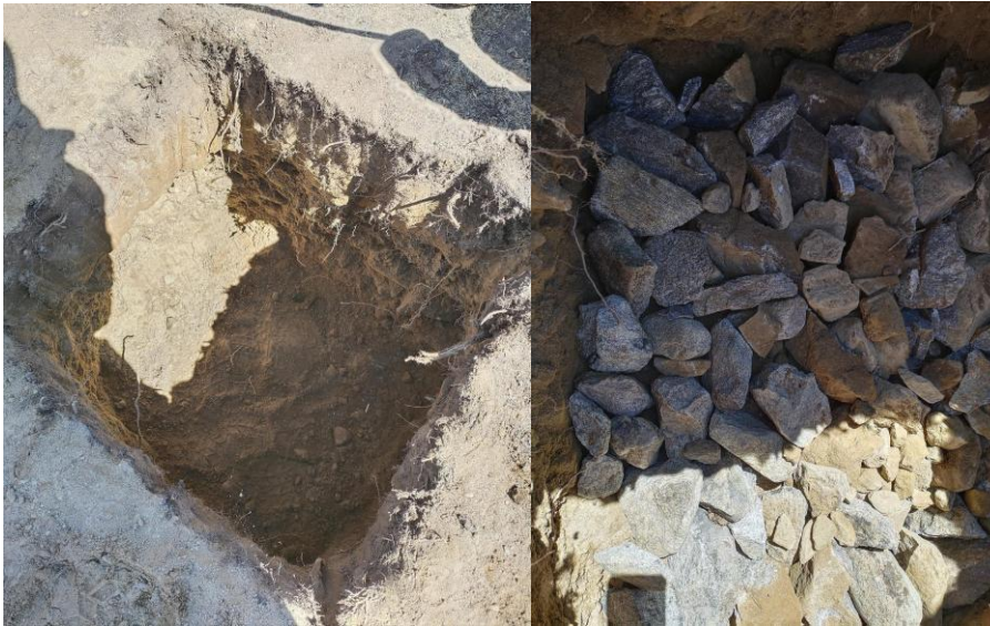
Figure 1:Left-Earthwork Excavation; Right-Hand-Packed Stone Soiling
