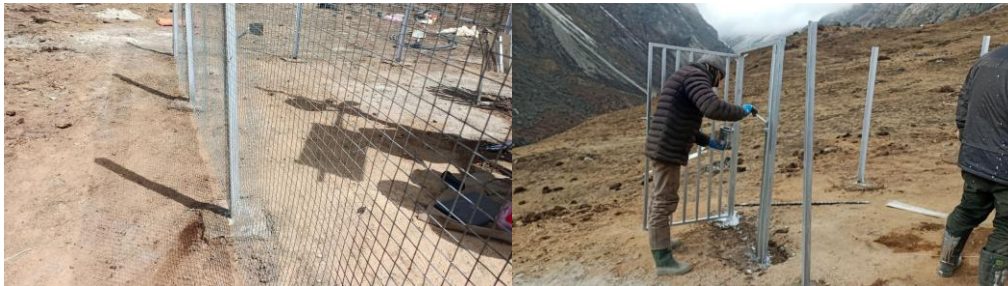
Figure 4:Left Side-Fencing work; Right Side-Applying aluminum paint
