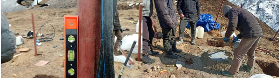
Figure 3:Left side-fixing centering; Right Side-Mixing Concrete
