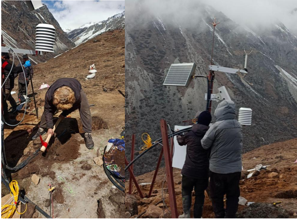
Figure 5: Left Side-Burying pipe underground; Right Side-Piping the wires
