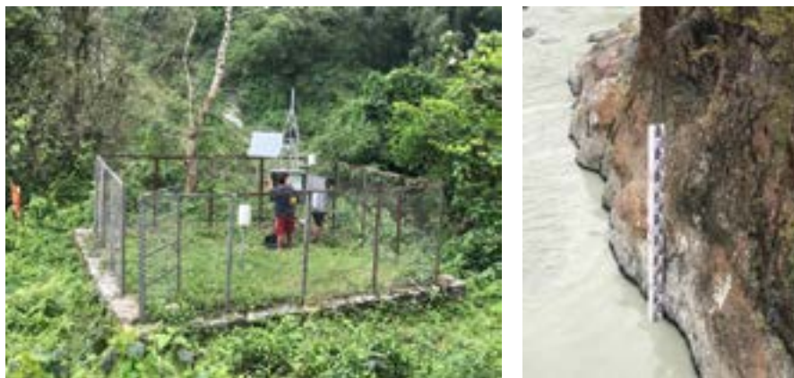
Figure 15: AWLS and new manual gauge station installation at Sadumadu
