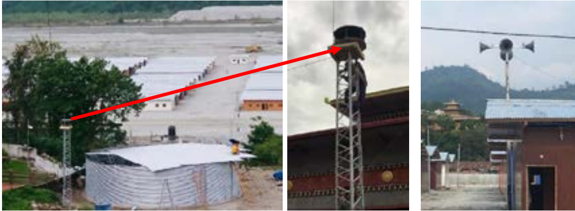
Figure 27: Siren installed for dissemination of flood warning information.
