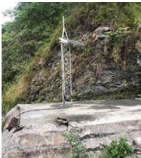
Concrete base near bridge for ALWS setup
