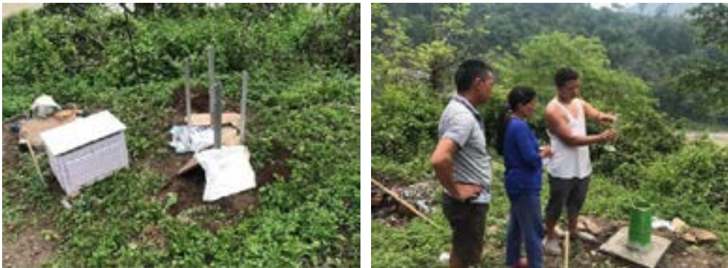
Figure 17: Installation of Class C station work and training site staff at Doyayang
