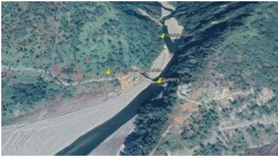
Figure 16: Location of Manual Class C station at Doyayang
