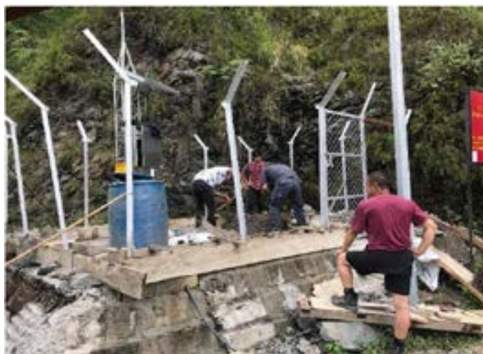
Field work for installation of AWLS at Doyayang
