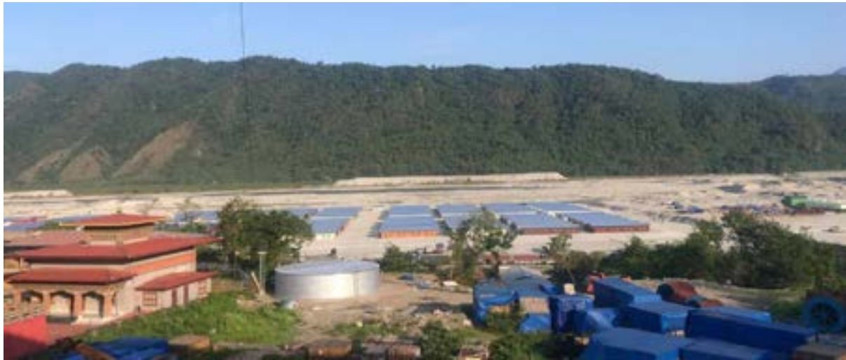
Figure 1: Temporary Shelter built at Amochhu bank, Phuentsholing
