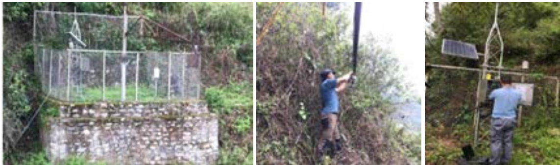
Figure 22: AWLS location and maintenance work at Sombaykha
