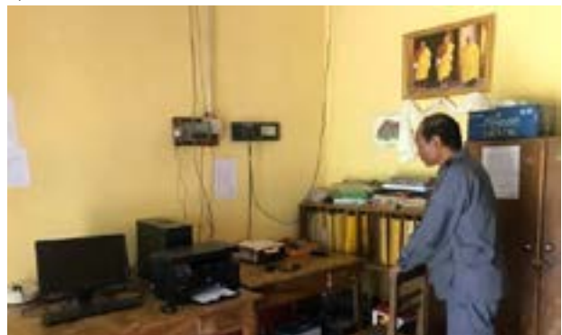
Dorokha HF Communication Room
