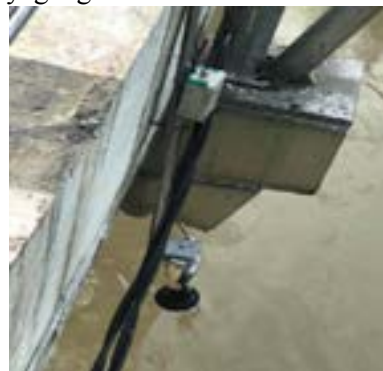
Radar sensor facing water placed on Amochhu Bridge
